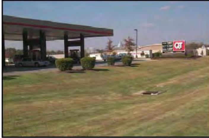
Description: Uniformly graded and densely vegetated sections of land engineered and designed to treat runoff and remove pollutants through vegetative filtering and infiltration.
