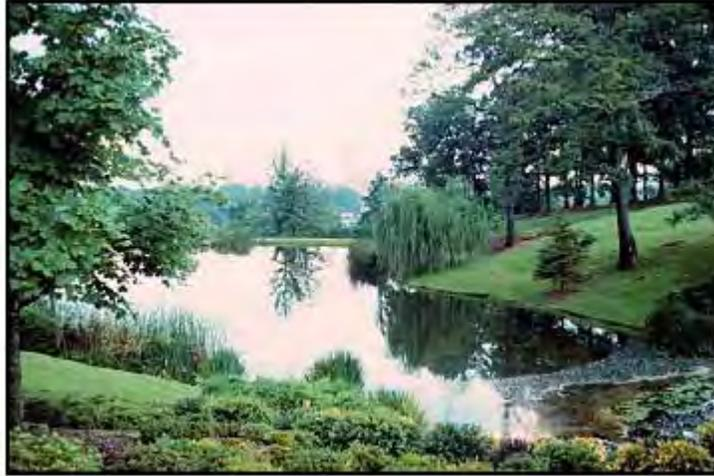
Description: Constructed storm water retention basin that has a permanent pool of water in which runoff from each rain event is captured and treated in the pool.
