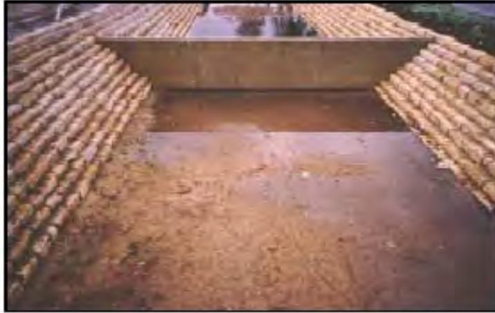
Description: Multi-chamber structure consisting of a pretreatment chamber, a sand bed as its primary filter media, and an underdrain collection system - designed to treat storm water runoff through filtration.
