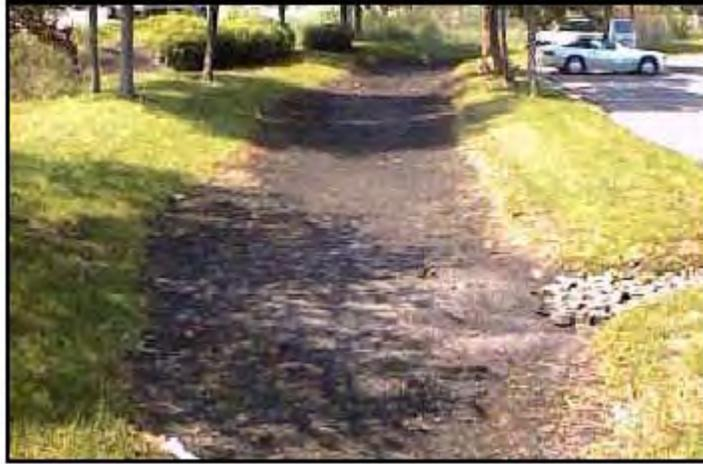
Description: Excavated trench filled with stone aggregate used to capture and allow infiltration of storm water runoff into the surrounding soils from the bottom and sides of the trench.
