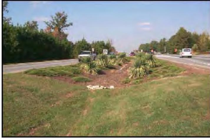
Description: Vegetated open channels that are explicitly designed and constructed to capture and treat storm water runoff within dry cells formed by check dams or other means.
